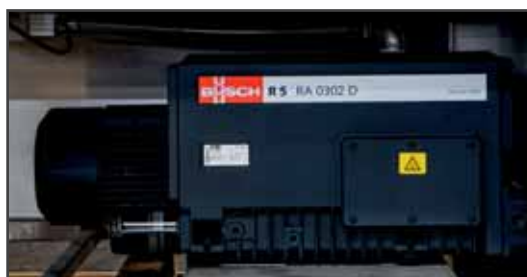
VP-900 TBA 300 & VP-1100 TBA 300 Pump 302m 3 /h
